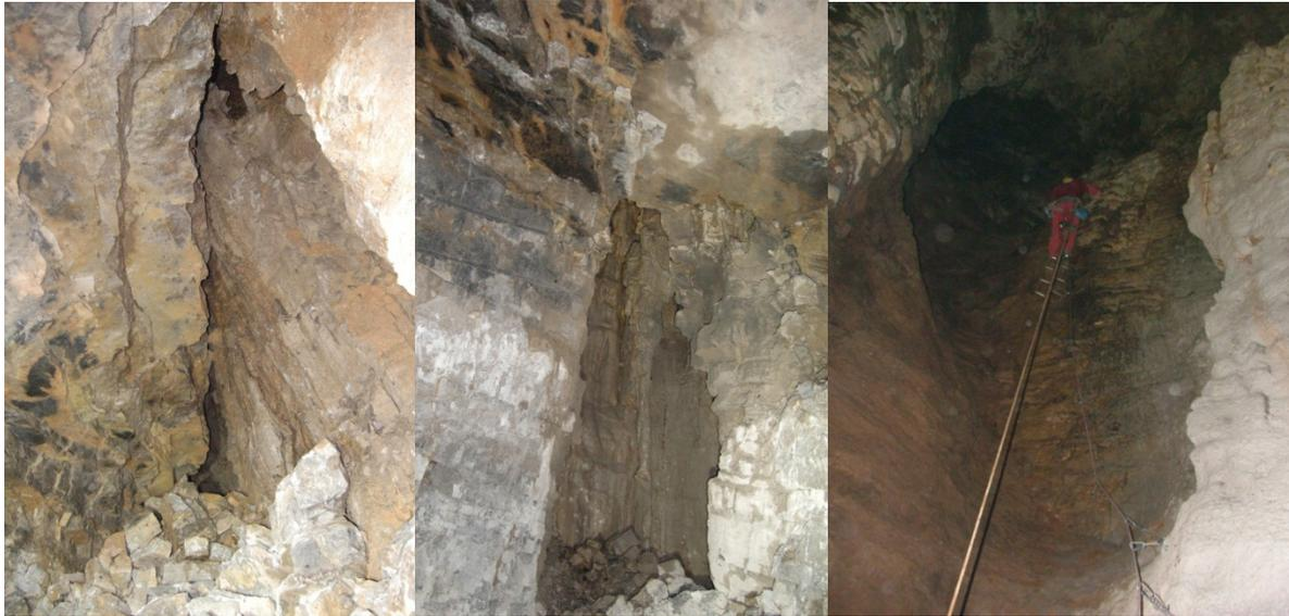
**Figure 6.** Views of the karst chimney encountered during excavation.
