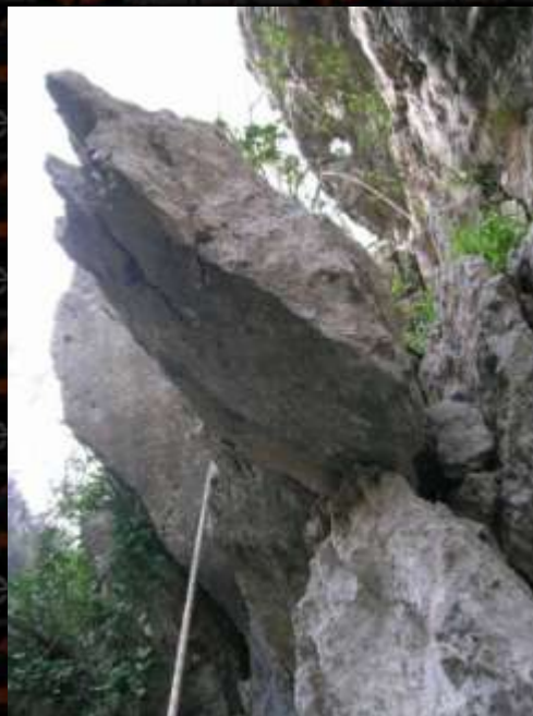
Flexural instability combined to presence of sub-vertical joints (type 3)
